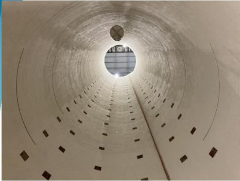
PM17 shaft final lining
