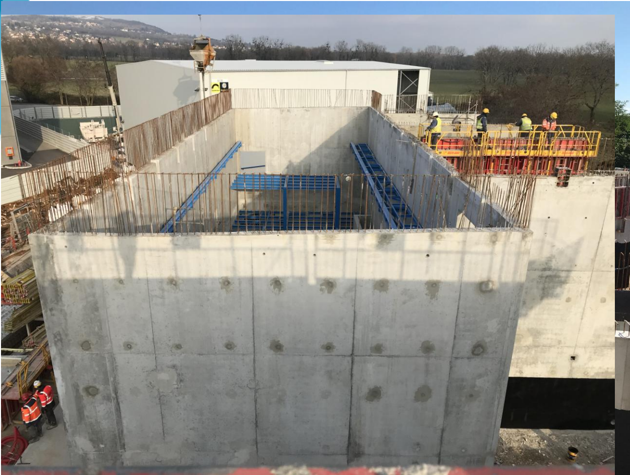
SF57: Wall casting
