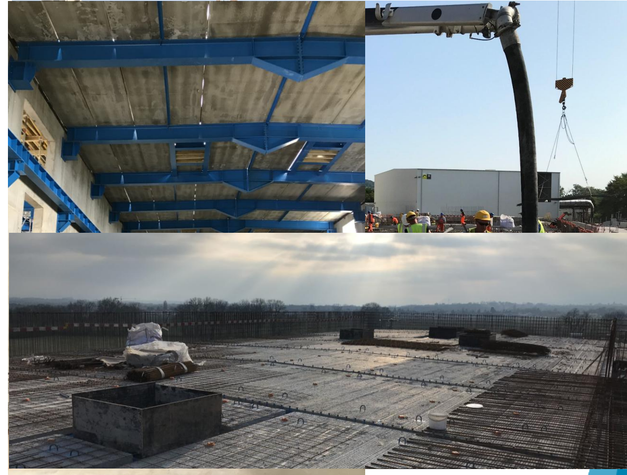
SHM57: Ground slab casting
